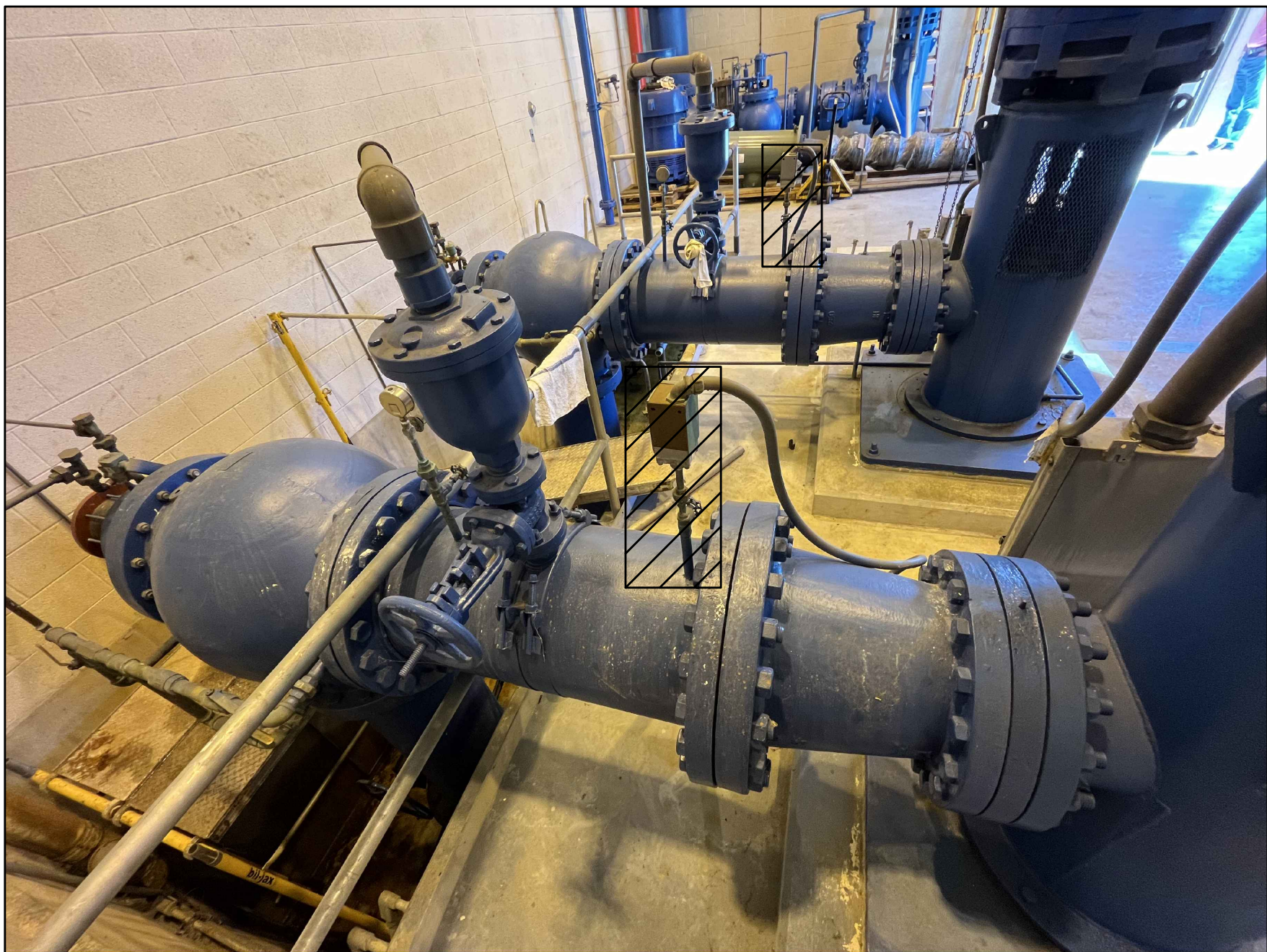
FINISHED WATER PUMP PRESSURE SWITCHES
